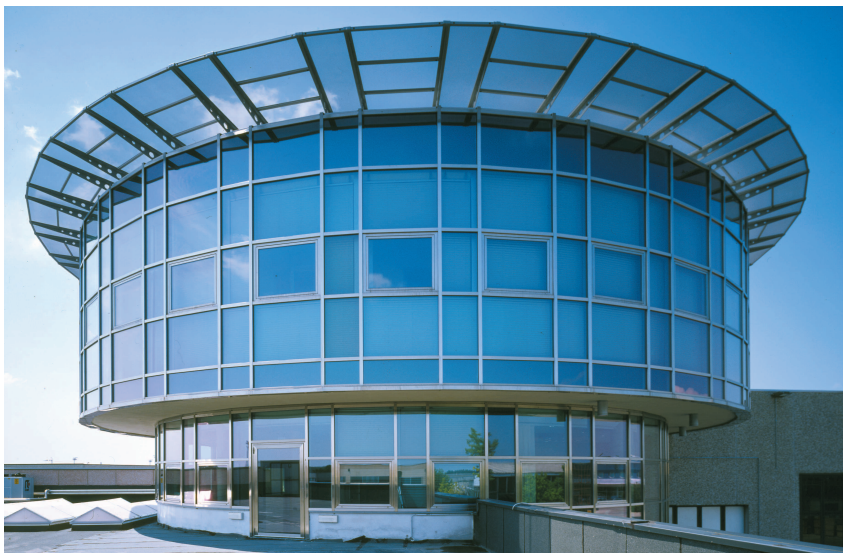
Fergamma Offices, Italy – Architect: Amerigo Berto
